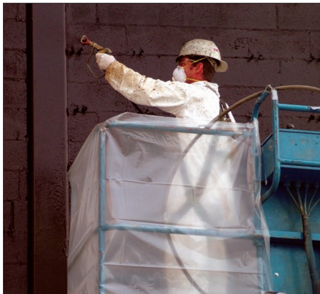
Water-based products are a safe choice for most applications, but require an ambient temperature at or above 0 C (32 F) to apply and cure. Where this is impossible, solvent-based products are sometimes the only solution.
