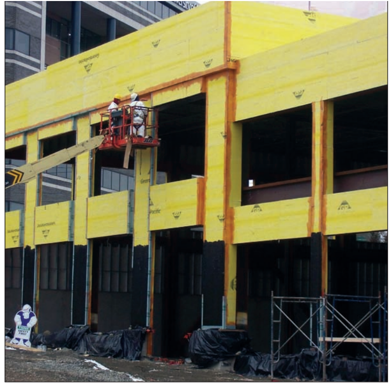
The percentage of solids in a vapour-barrier can vary, but contrary to popular belief, a higher solids-content does not necessarily mean a better product.
